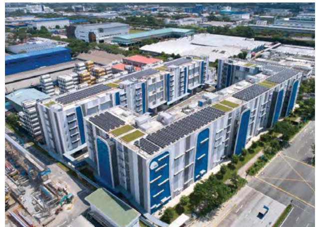
SolarRoof installation on JTC Space @ Gul. Image: JTC.
