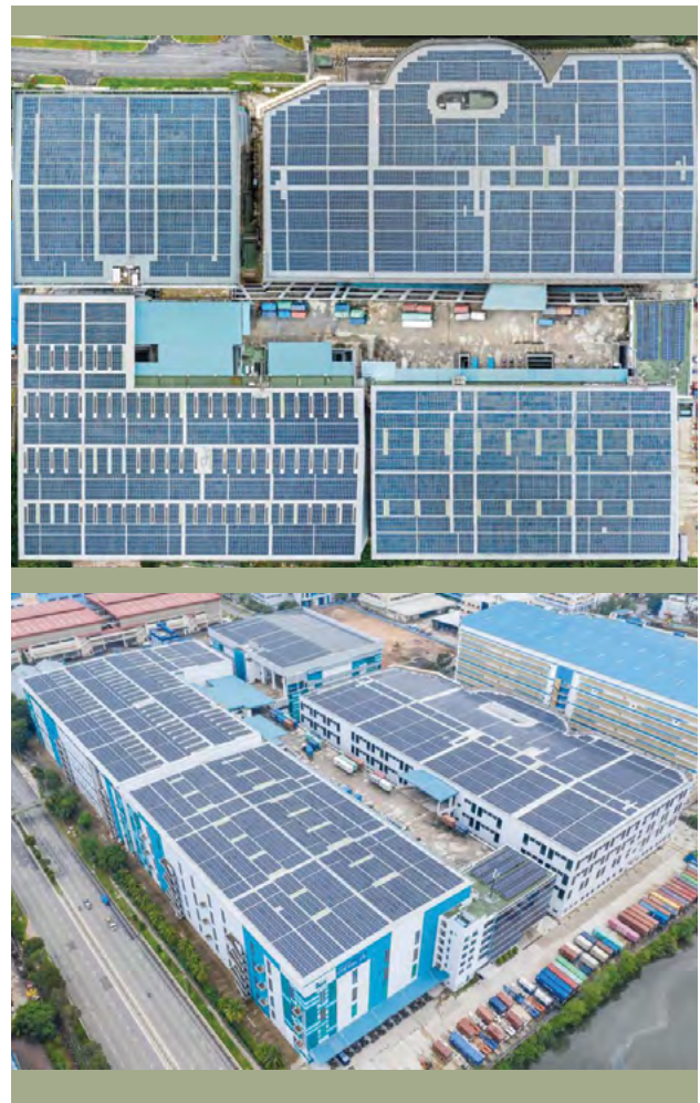
Solar installations at 40 Penjuru Lane. Images: CapitaLand and Sembcorp.
