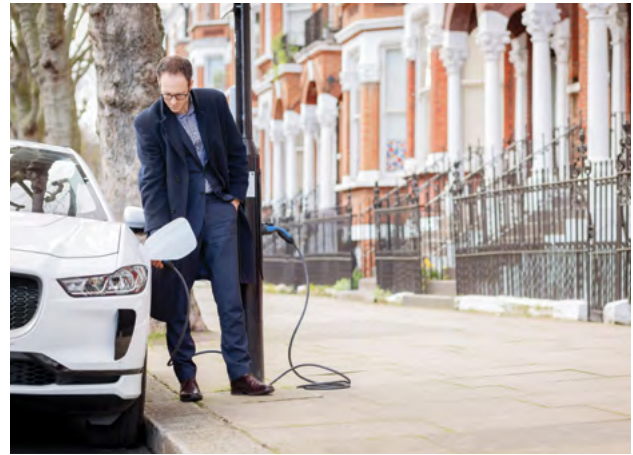
Sutherland Avenue is UK's first residential avenue fully converted to provide lamp post electric vehicle charging points.
