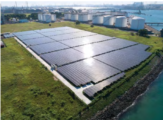
SolarLand installation on Jurong Island. Image: JTC.
