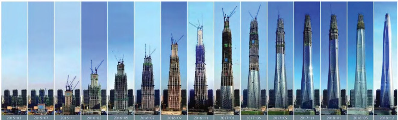
Time-lapse photo collage showing the construction sequence, from basement, superstructure, facade and internal MEP system, to completed project. Image: CSCEC.
