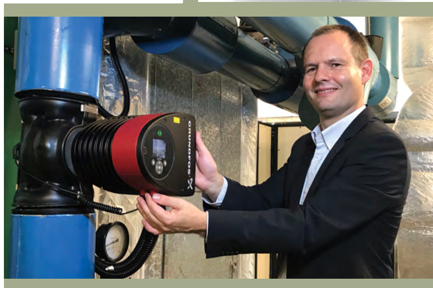
Mr Anders Christiansen, Regional Business Director, Building Services, Grundfos Asia Pacific with the Distributed Pumping System installed in the cooling circuit.
