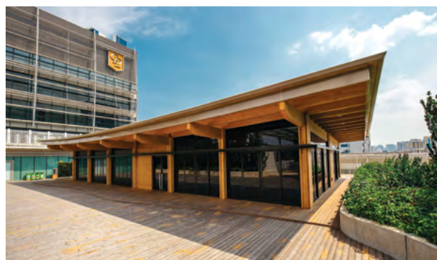
The Singapore Sustainability Academy is one of CDL's sustainably designed and built projects. Located at City Square Mall, Singapore's first Eco-mall, the zero-energy academy is a Green Mark Platinum building awarded by the Building and Construction Authority, and the first in Singapore to have its construction materials, Cross Laminated Timber (CLT) and Glued Laminated Timber (Glulam), verified by the Nature's Barcode system as coming from responsible sources.
